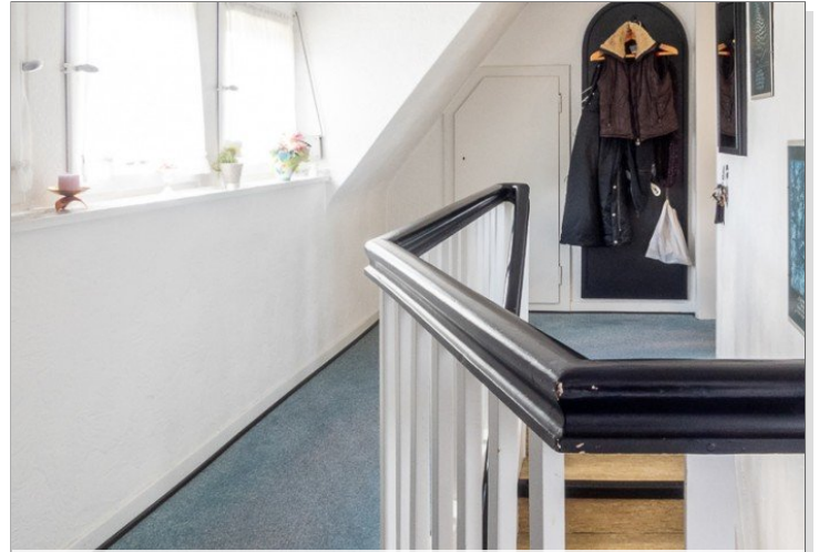
9586DG Flur -Altbau-
